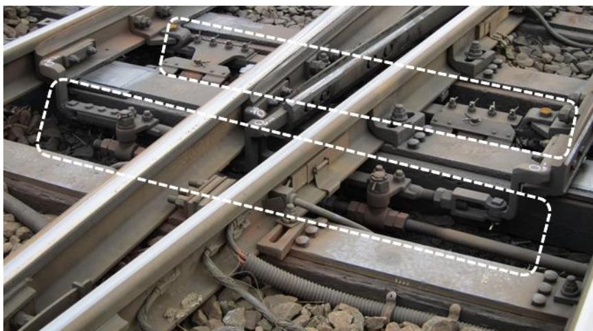
Fig. 6.3 Picture of the toe of tongue rail (measured double slip switch).
